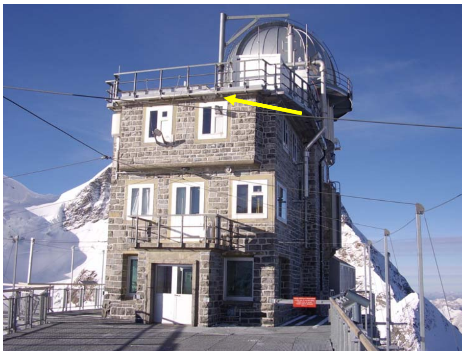
Fig. 2 “Sphinx”-station on the Jungfrauoch (northeast side). The external sampling unit of the LOPAP instrument is shown by the yellow arrow.
