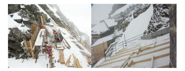
**September:** At the moment, there is construction work going on at Jungfraujoch, as the research station is getting a new protective roof. In the future, the new, steeper roof should prevent the accumulation of too much snow. Due to the bad weather this summer (lots of snowfall), work at this height is even more difficult and rather slowly progressing.
