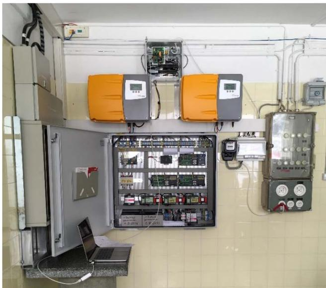
Figure 5. New fast data logger for noise detection mounted above the two PV inverters at Jungfrauoch.
