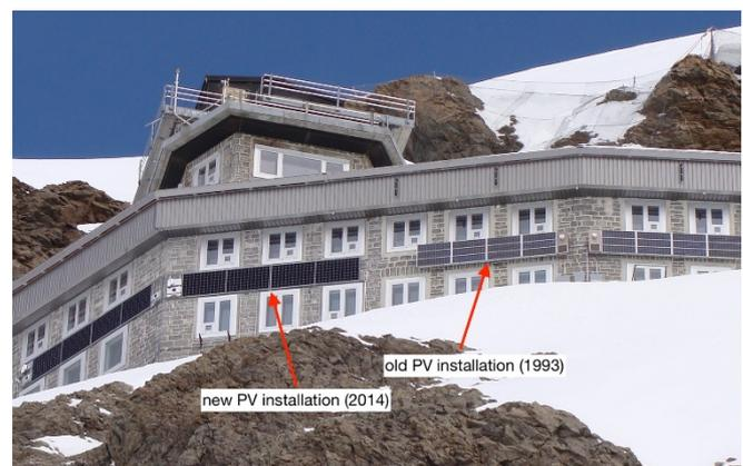
Figure 1. New (2014) and old (1993) PV modules installed on the façade of the Jungfrauoch building.
