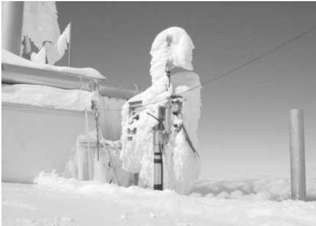
This picture taken on September 17, 2001, at the top of the Sphinx Observatory shows the 70cm corner-reflector (below) and the 23cm hybrid-quad antenna (above).
