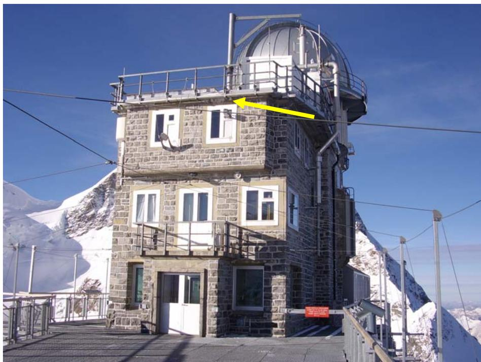
Fig. 2 “Sphinx”-station on the Jungfrauoch (northeast side). The external sampling unit of the LOPAP instrument is shown by the yellow arrow.
