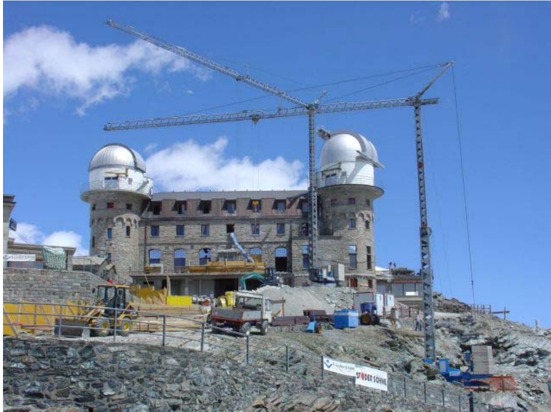
July: Construction site at Gornergrat.
