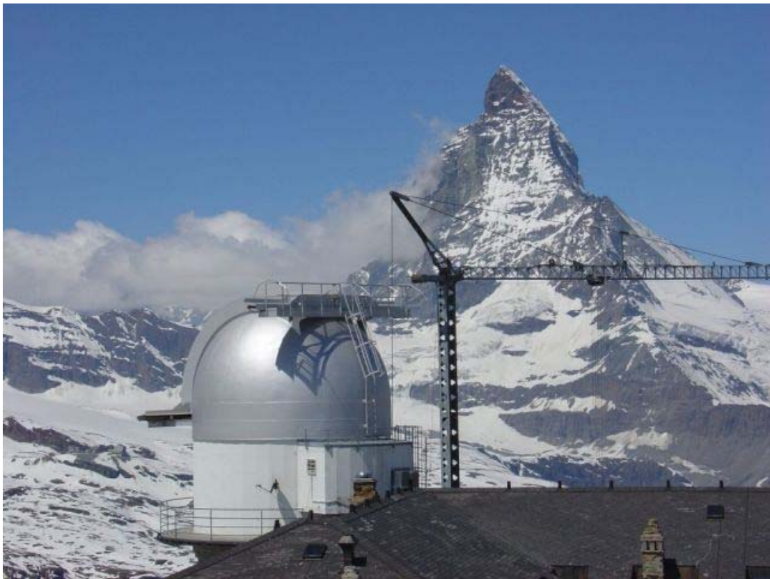
October: Construction scene at Gornergrat.
