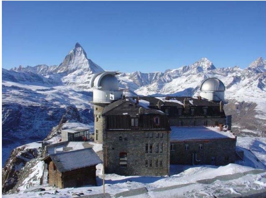
January: Reopening of Kulm Hotel and the renovated astronomical observatory Gornergrat South.
