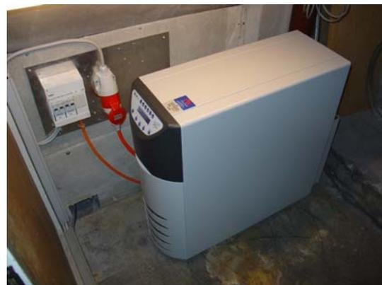
**Figure 6:** The new central UPS in the Sphinx laboratory
