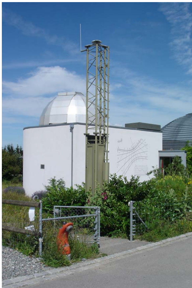
Fig.1: The successful replacement of the antenna at the AGNES station Kreuzlingen
