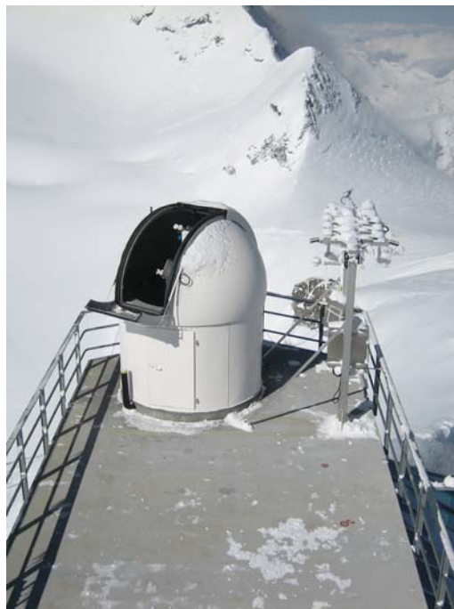
Figure 3: Solar radiation measurement deck
