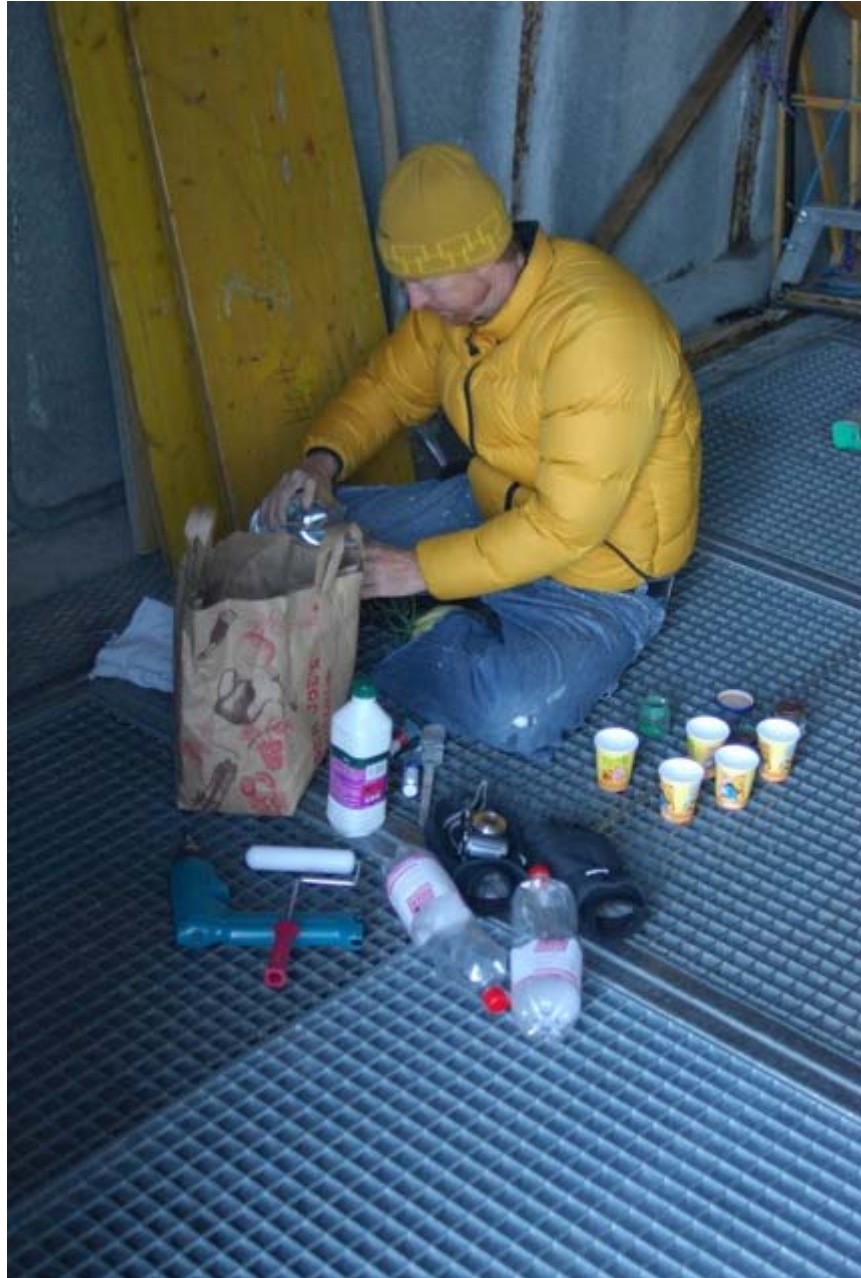
Mixing paint at high altitude.
