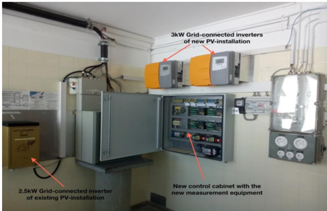
Figure 2. The two new grid-connected inverters and the new measuring equipment.
