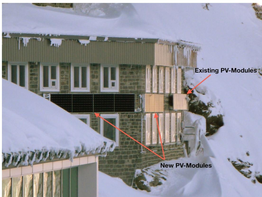
*Figure 1. The extension mounted at Jungfrauoch in 2014 with new PV modules on the south and southwest wall (installations on the left) is located near the already existing PV installation from 1993 with 1'152 Wp (installation on the right).*
