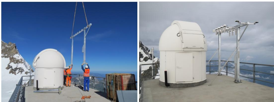
*Figure 1. Installation of the new measurement bench on the Sphinx terrace (left) and Jungfraujoch SACRaM station after completion of the renewal. The new measurement bench holds more available positions than the previous one, and all cabling are now located within the metallic structure and are thus protected from the harsh meteorological conditions.*
